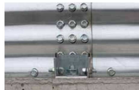
Intermediate base anchors allow single pass unloading in large Sukup Bins.
