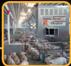
The inside mount model is a gas circulating heater ideal for a confinement environment.
