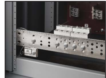
Fig. 17: Ground and neutral disconnect links
